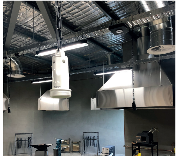
Hyena suspension sockets are used to provide pendant power for textile cutting and metal engraving.
