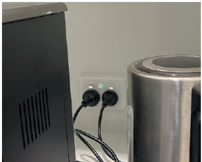
Powermesh DGPO LED flashes green when high energy appliances are in use.
