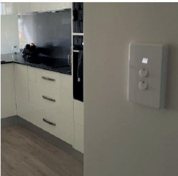
Manual override created in the downstairs hallway using 2 buttons.
