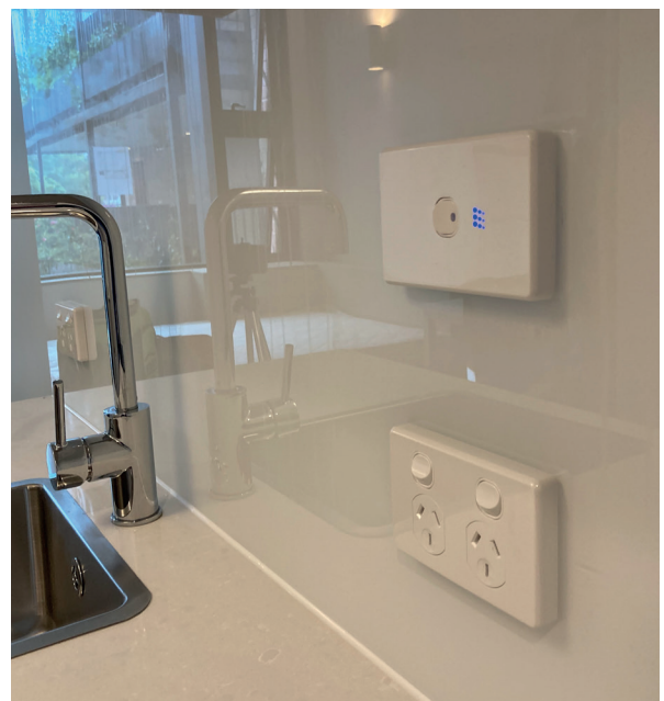
Powermesh Connected Home Multi-Purpose switch wired to the cooktop
