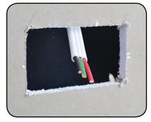
Trace around the rear of the wall box against the wall and cut out the aperture to fit the box. Ensure to cut cleanly so that the box is a neat fit.
