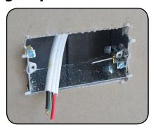
3. Once assembled through the aperture spread the flap outwards.
