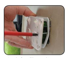
In order for wall box to achieve acoustic rating, ensure that supplied gasket is neatly sandwiched between wall plate and plasterboard during fastening of 84mm mounting screws.
