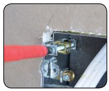
5a. Push the locking tabs outward, ensuring the screw assembly is aligned and fasten until the tabs lock the box into the plasterboard.
