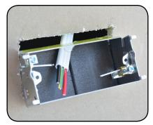
2. Place cables through the relevant cut out feature, trying to keep others sealed and insert the box through the opening, squeezing if necessary.
