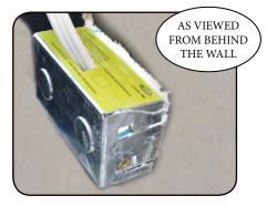
4. Ensure the box fills the aperture and is pushed back on the tags correctly.
