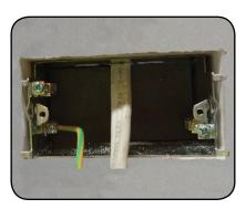
Box has been tested and is capable of withstanding FRL-/120/120 without fire rated mastic (EWFA Report No. 47083900.01). Ensure intumescent foam pads supplied are correctly positioned at rear of box to enable fire rating to be achieved.
