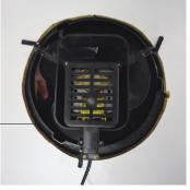
Assemble fan frame through ceiling hole. Plug into socket ensuring power is off. Tighten screws and ensure clamp plugs are securely positioned.
