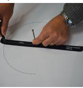
Use Cutting Template found on the Cut out the hole using box lid to mark the cut out. plasterboard saw.
